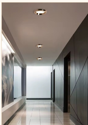
Adjustable downlights, corridor scheme
