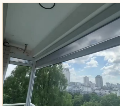
Motorised zip screen, high-rise balcony
