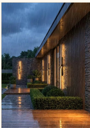
Exterior linear wall lighting
