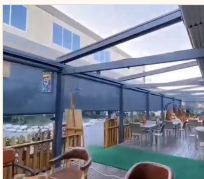
Glazed pergola enclosure, restaurant terrace
